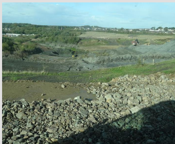
"The Seiont Quarry in October 2019 during a visit by NWGA to the Caernarfon By-pass groundworks by invitation of Jones Bros Civil Engineering UK", image by Lyn Relph.
